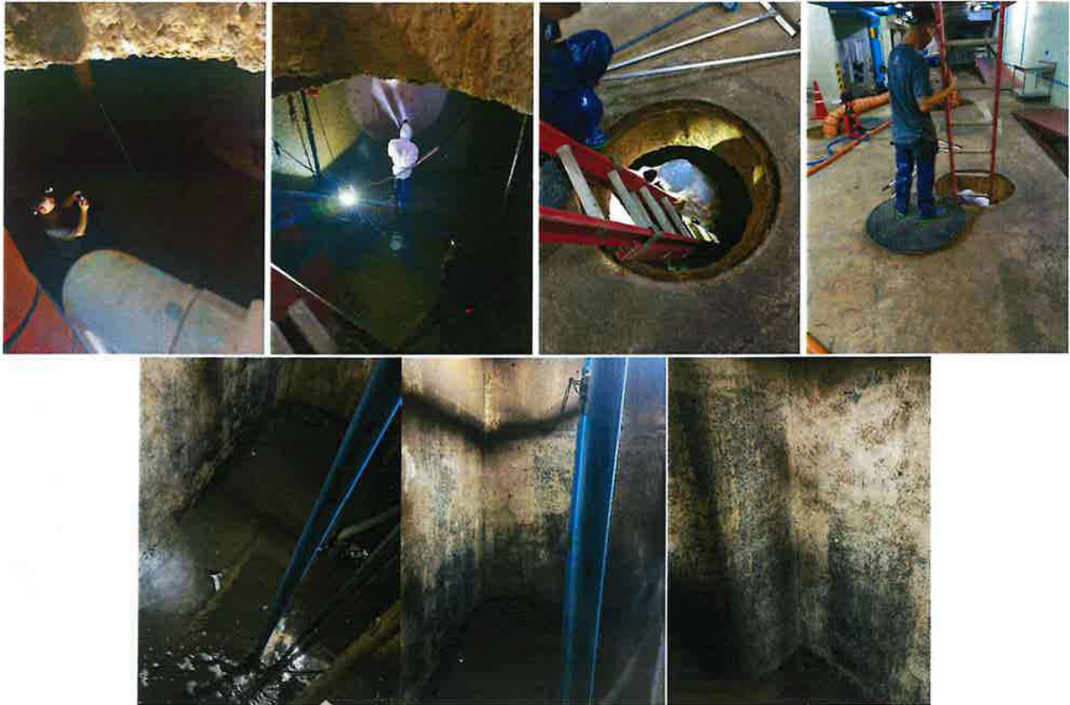
Photo - Cleaning sludge tank
